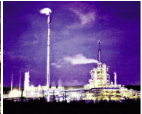
▲ Wabash River Coal Gasification Plant
