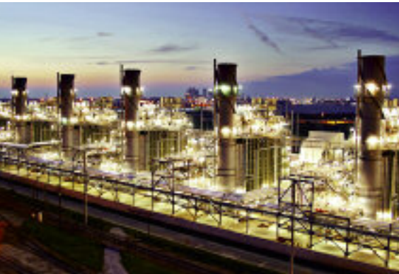
▲ Tampa Electric's Polk Power Station
